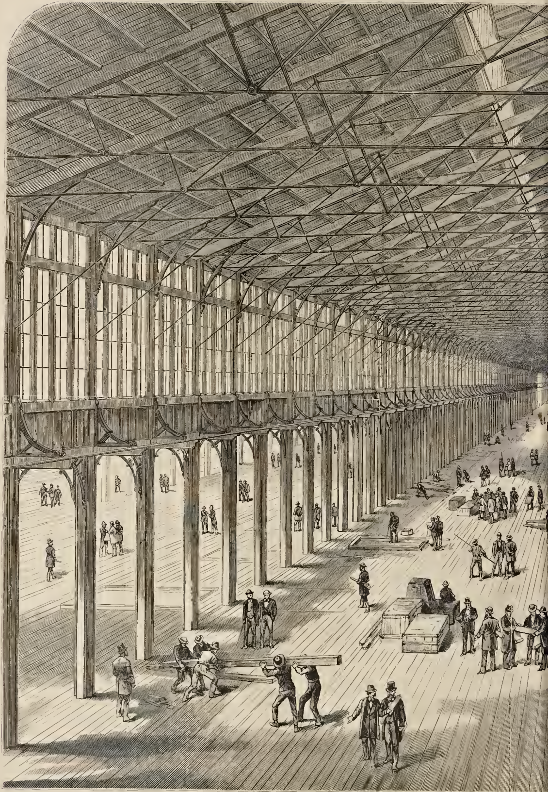
INTERIOR VIEW OF THE MACHINERY BUILDING, WHILE IN PROCESS
