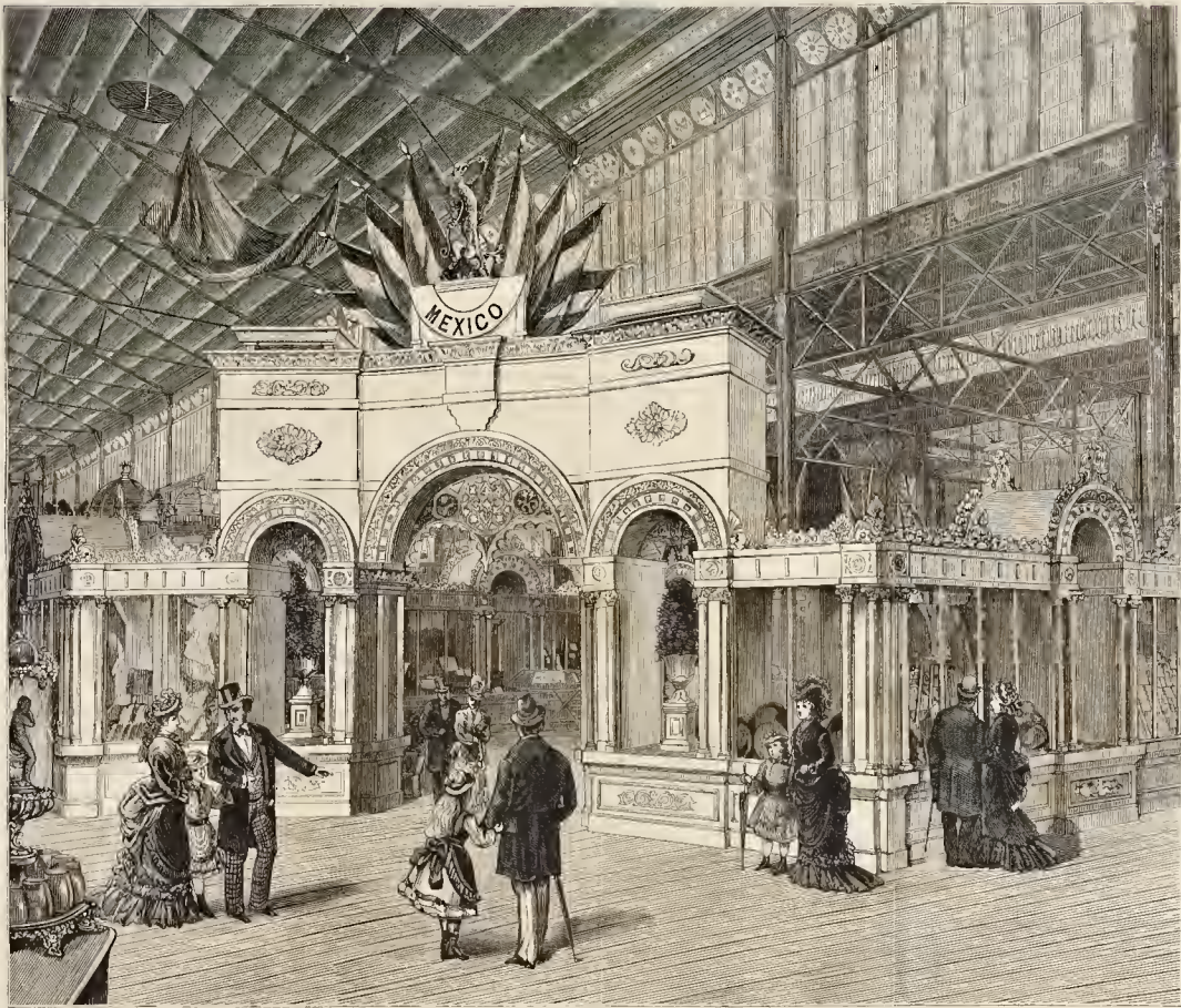
MEXICAN SECTION, IN THE MAIN BUILDING.
