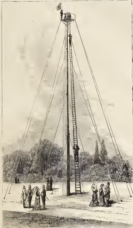
DAVIS ELEVATING SIGNAL-TOWER.
