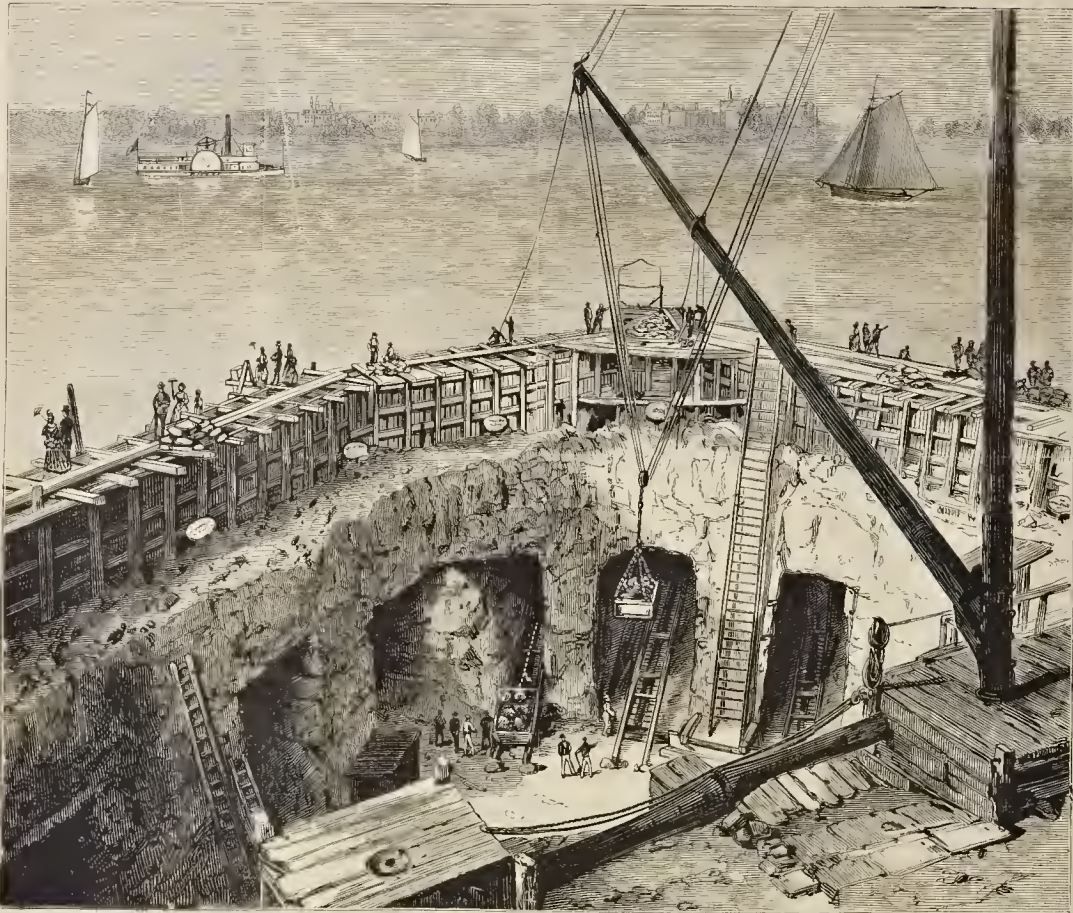
COFFER-DAM AND ENTRANCES TO THE AVENUES EXCAVATED THROUGH THE SOLID ROCK AT HALLETT'S POINT.
