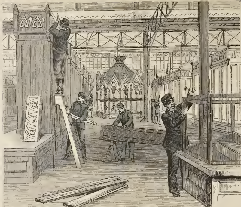
CONSTRUCTING THE CHILLAN COURT IN THE MAIN BUILDING.
