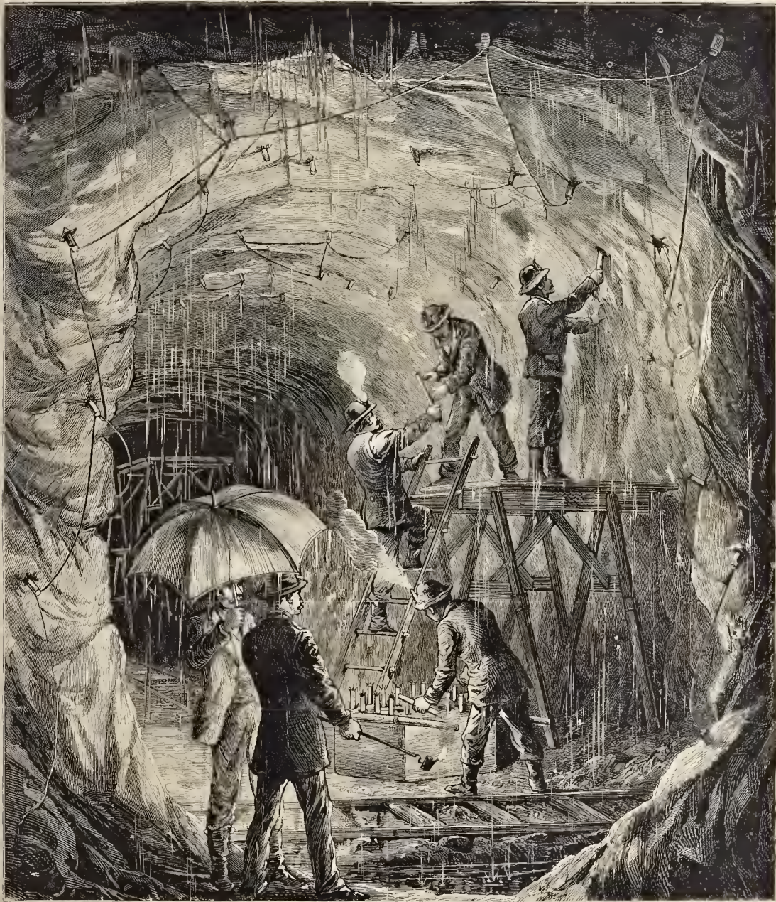
THE GREAT BLAST AT HELL GATE—CHARGING THE ROCKS OF THE SUBAQUEOUS MINE WITH CARTRIDGES OF NITRO-GLYCERINE.
