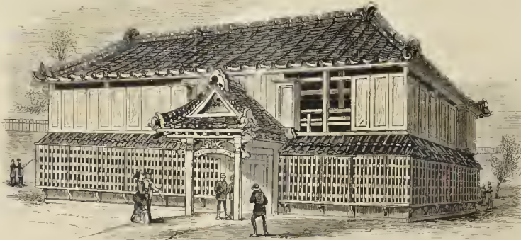
HEADQUARTERS OF THE JAPANESE COMMISSION, ERECTED BY NATIVE WORKMEN.
