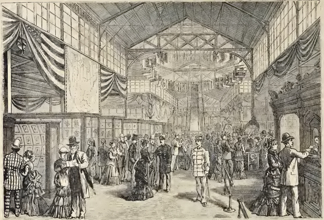
INTERIOR VIEW OF THE POST-OFFICE AISLE.
