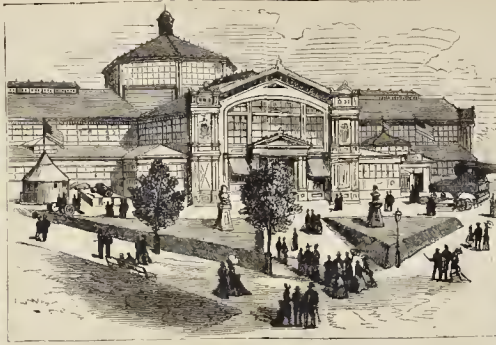
EXTERIOR VIEW OF THE UNITED STATES GOVERNMENT BUILDING.
