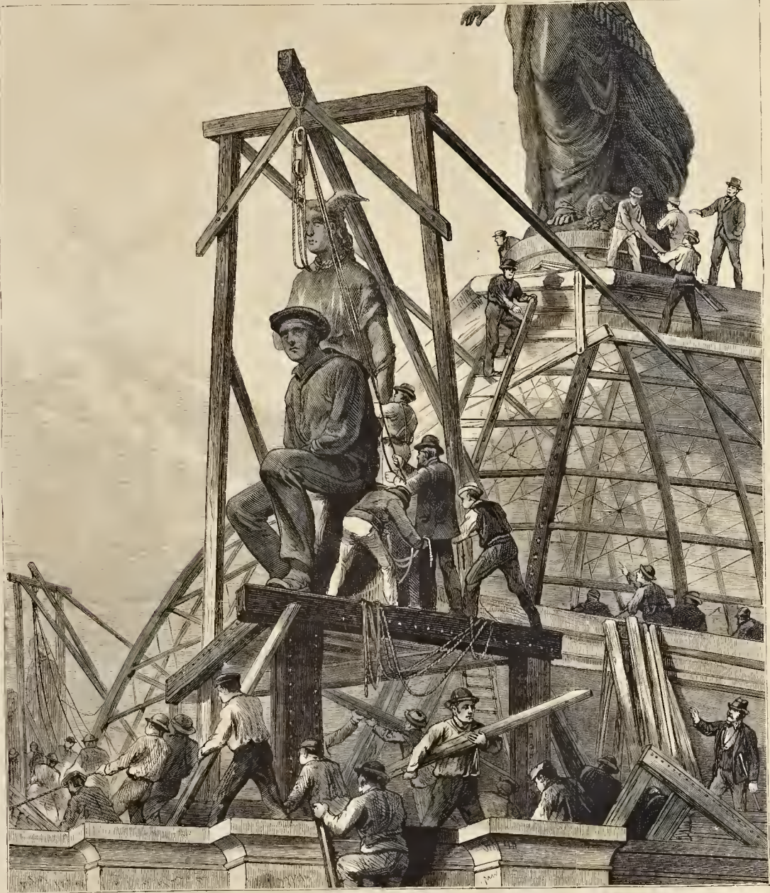
PLACING COLOSSAL STATUES AT THE BASE OF THE DOME OF MEMORIAL HALL.
