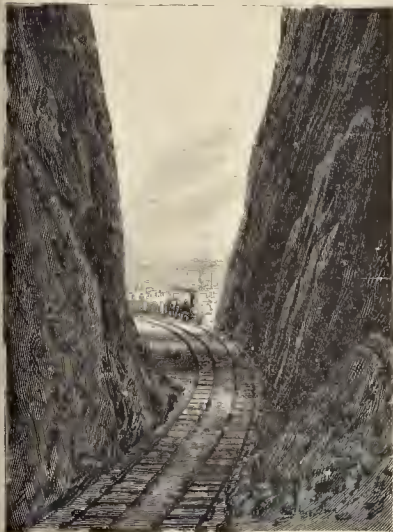
THE DEEP CUT AT BERGEN HILL, NEAR JERSEY CITY.
