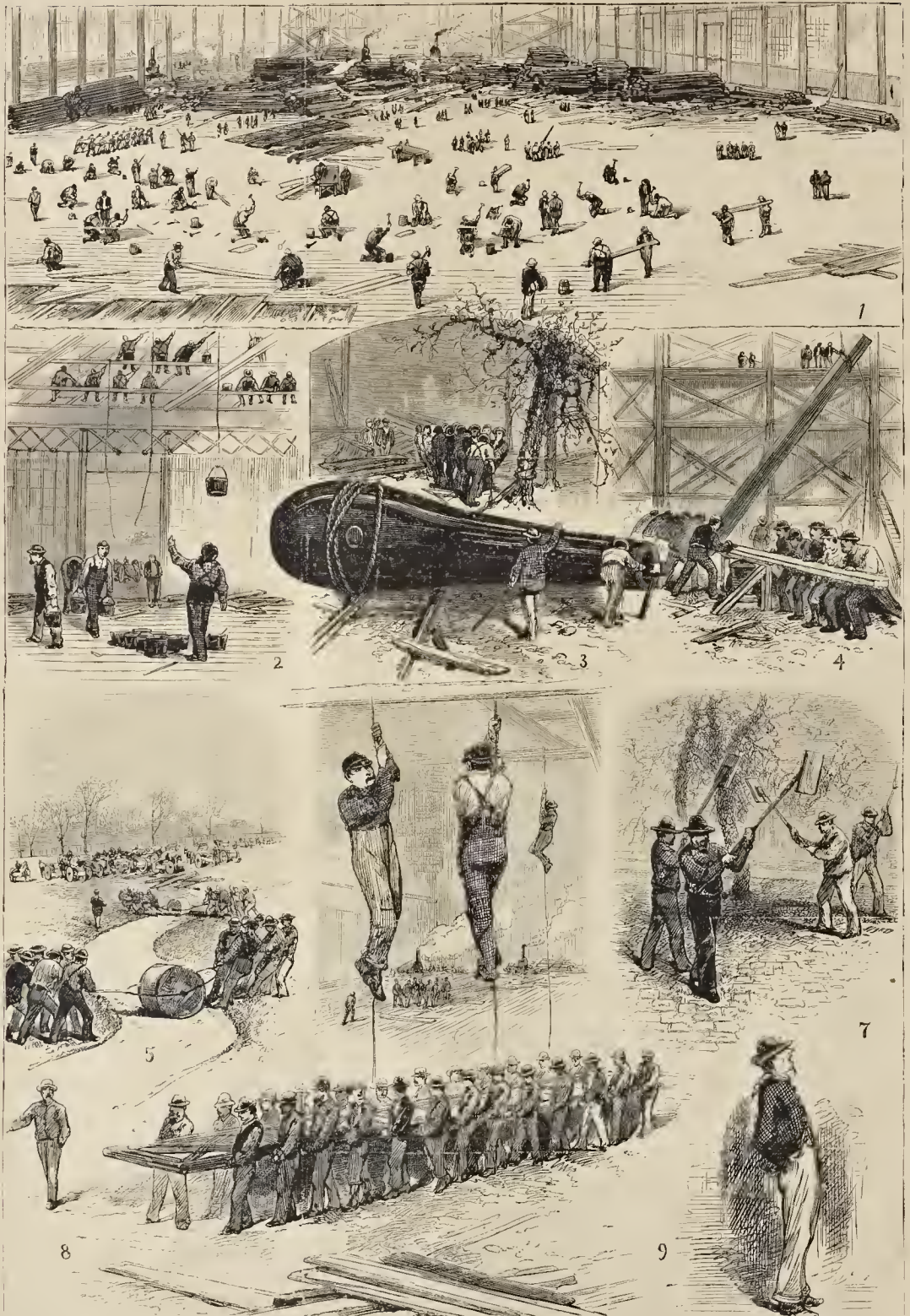
1. Carpenters flooring the Main Building. 2. Painters at work in Machinery Hall. 3. Arrival of a motor gun for the Government Bull Ring. 4. Hoisting a girder in the Main Building. 5. Making coal is on the Centennial grounds. 6. Workmen coming down to dinner. 7. Scaffolding the grounds around Horticultural Hall. 8. Carrying a girder to the transept of the Main Building. 9. A Centennial "loss."
