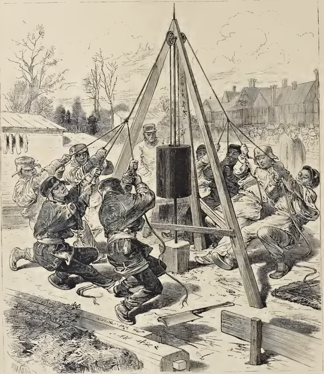
JAPANESE WORKMEN LAYING THE FOUNDATION OF THE JAPANESE BUILDING.
