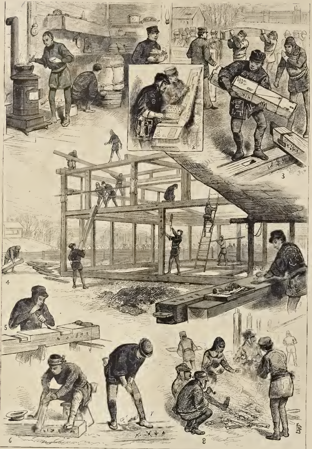
1. Japanese workmen preparing their meals. 2. The chief workman and his assistant consulting their books and charts. 3. Bringing joists and timber from Machinery Hall. 4. Erecting the Japanese dwelling house. 5. Mortising. 6. Sawing. 7. Using the adze. 8. Around the fire.
