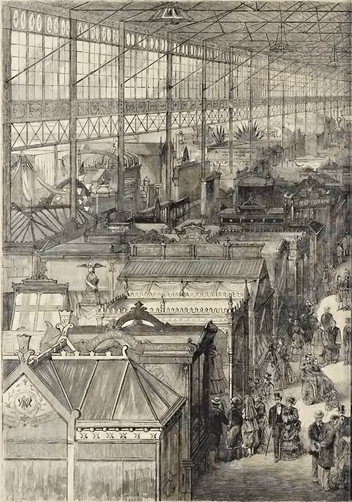
VIEW OF THE MAIN BUILDING, LOOKING DOWN THE CENTI
