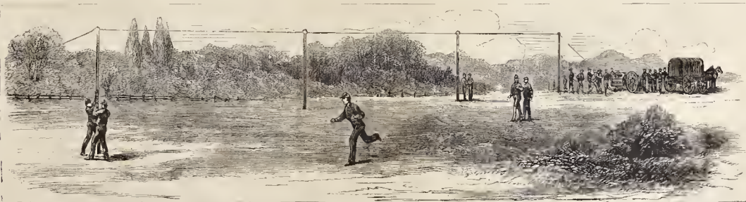
LAYING THE TELEGRAPH.
