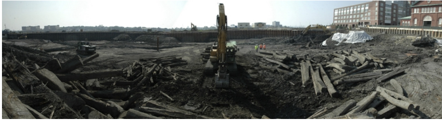
Fig. 1. Photograph of the timbers at Charlestown Navy Yard (Courtesy C. Taylor).
