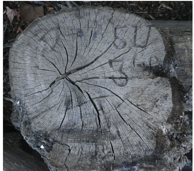
Fig. 5. Log mark stamped or hammered into a beam end, reading “5U 340” (authors).
