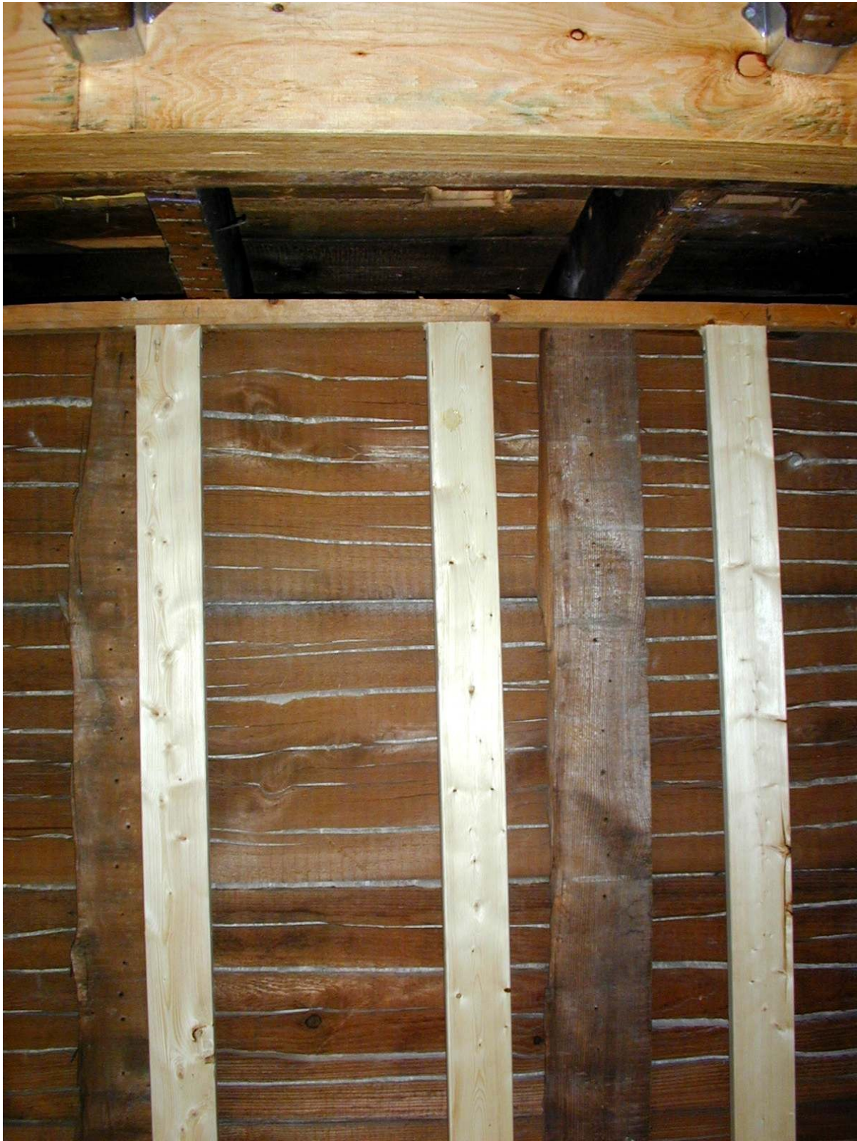
(F.) Hemlock split-board lath and oak ceiling joists in #929.
