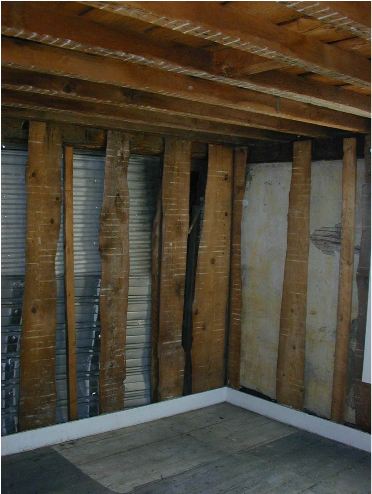
(D.) Slab wood wall studs cut in 1849 in the east room of #925.
