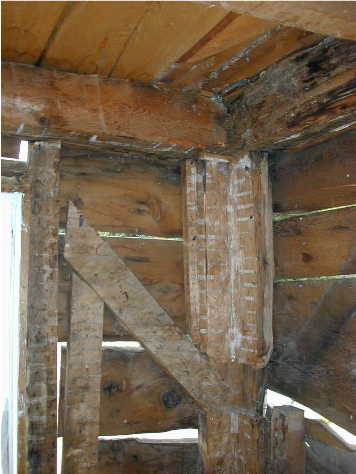
(E.) Re-worked corner post and wall bracing in older section of #925.
